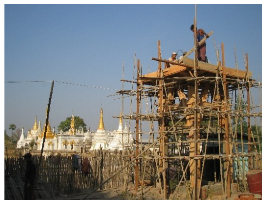
The new water tank under construction
