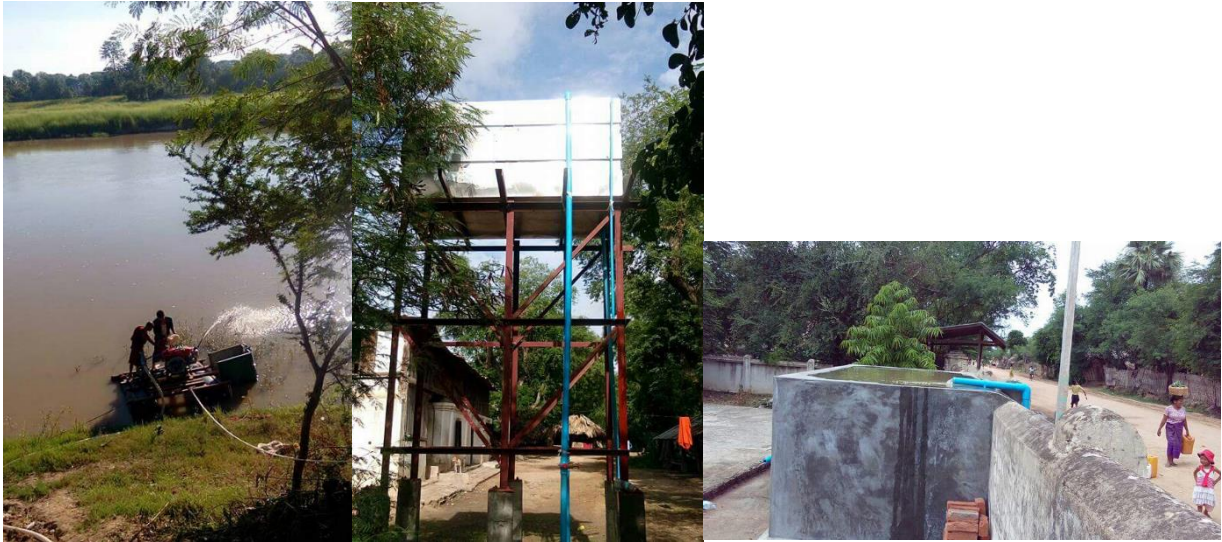
Pumping the water from the Mu River ... to the water tower ... and releasing it to the water stations in the village
